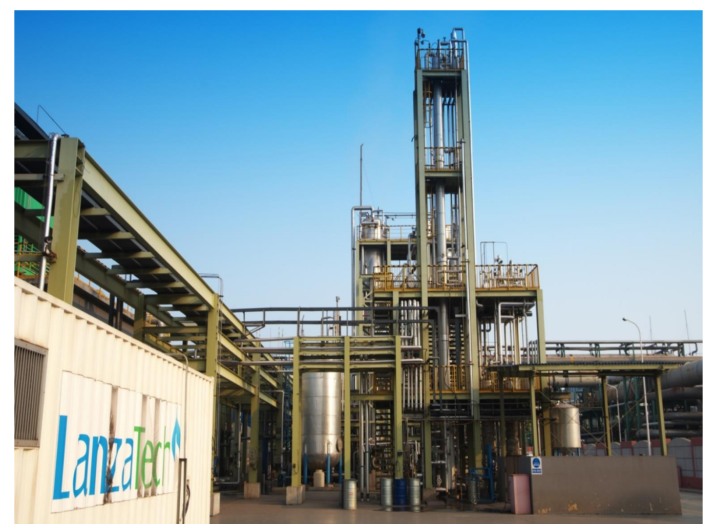
LanzaTech waste gas to fuel demonstration plant at Shougang Steel Mill
